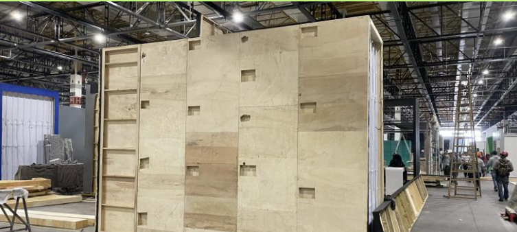
Stock panels with sheets on both sides and access ports for fixings
